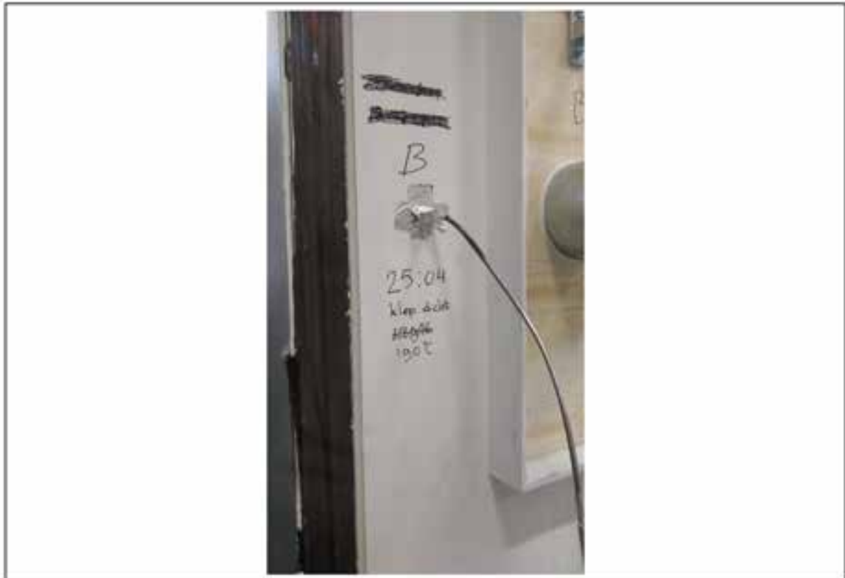
Photo C. 5: Closing time damper B
