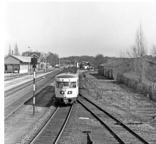
Emplacement station Doetinchem, 1978.
