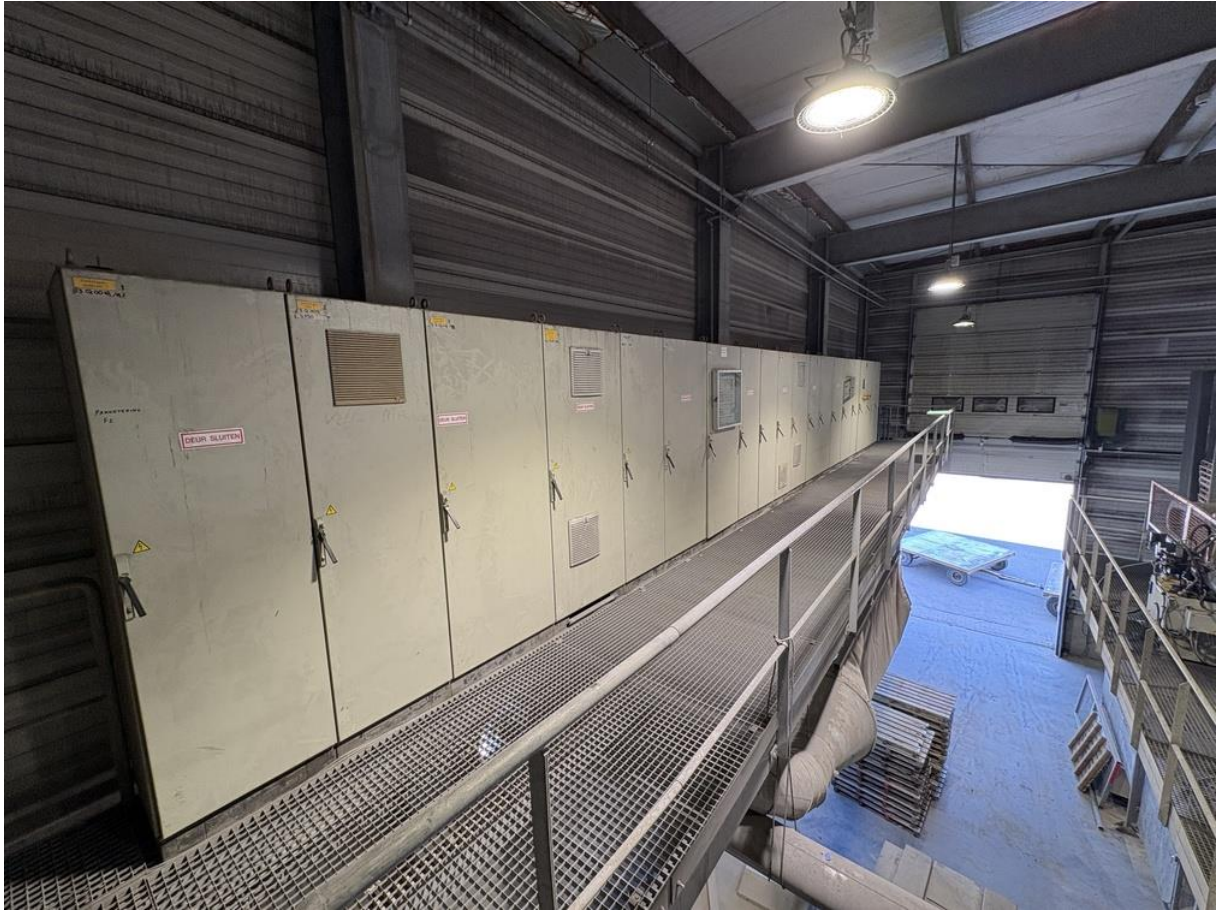
Control cabinets for packing line
