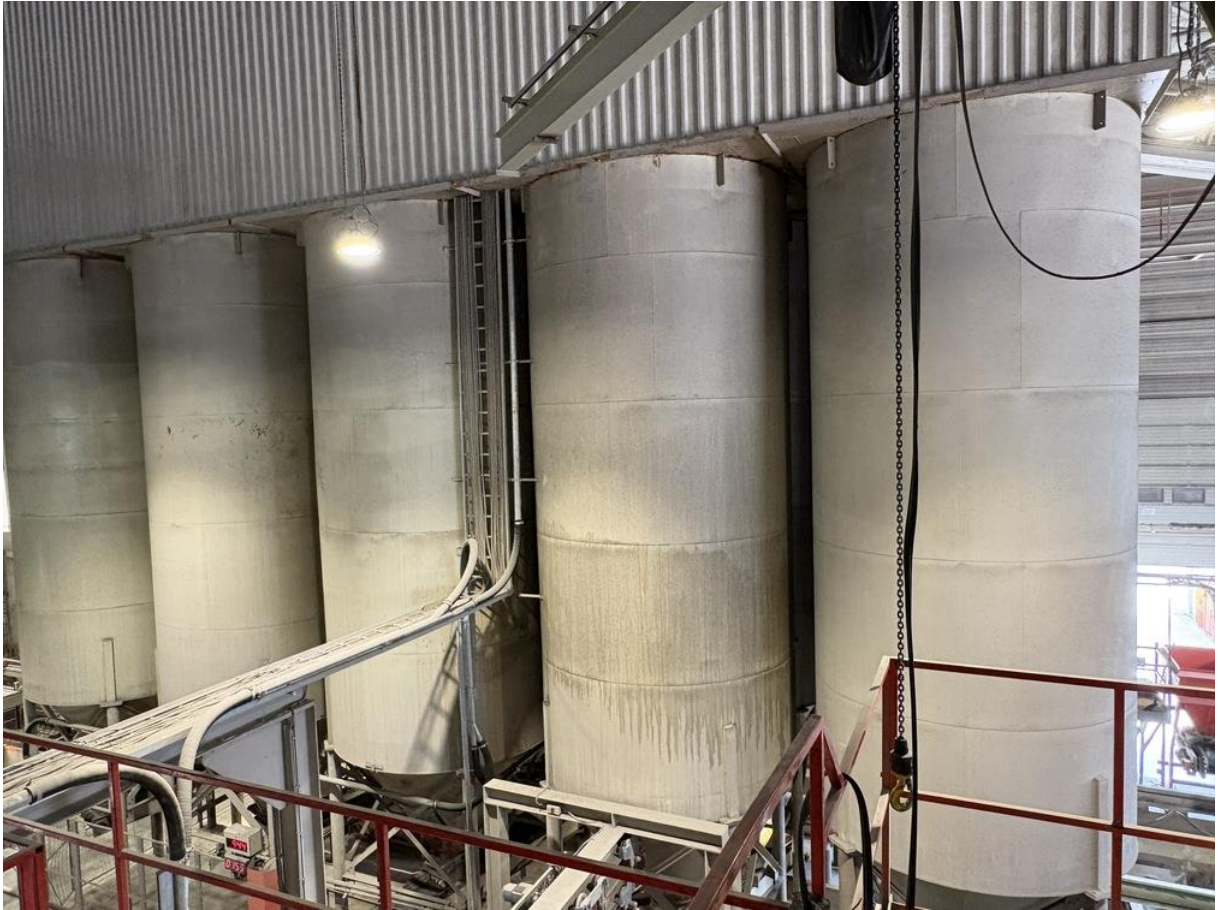
20 Storage silos for sand and aggregates
