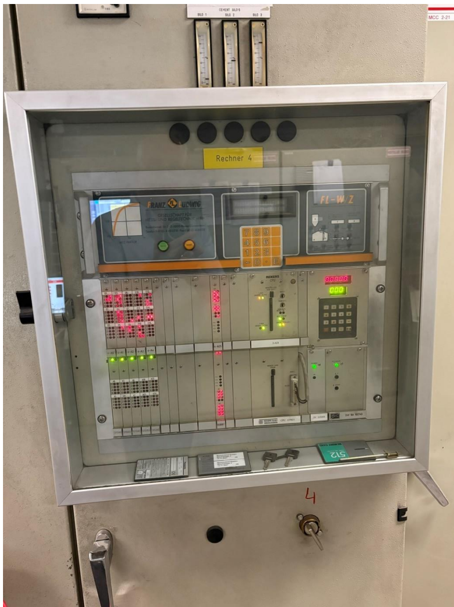
Ludwig water measuring and dosing Vibro 1
