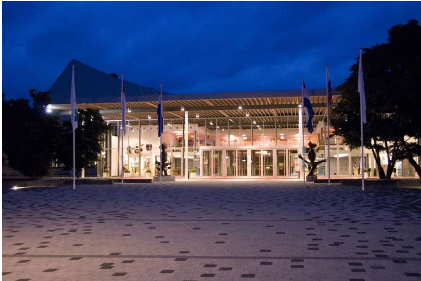
The renovated Rodahal
