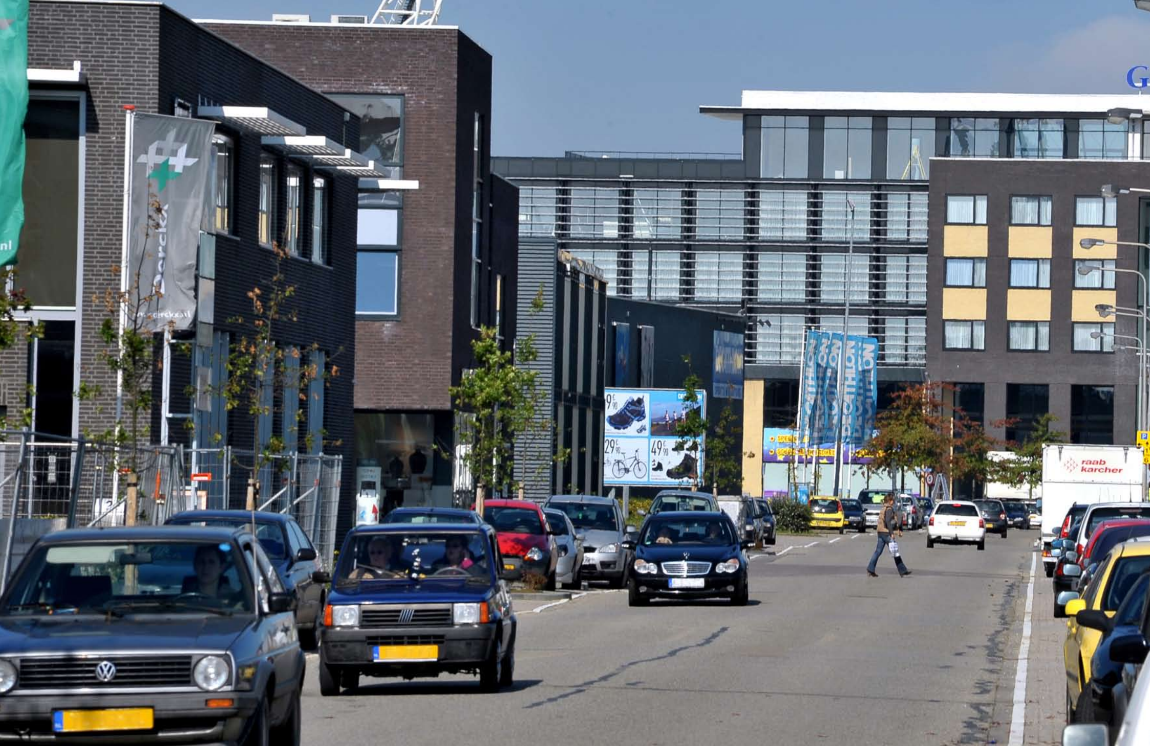
Rodaboulevard industrial estate
