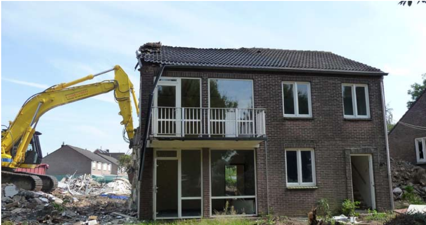
Demolition of semi-detached house at corner of Kommerveldlaan and Laurastraat
