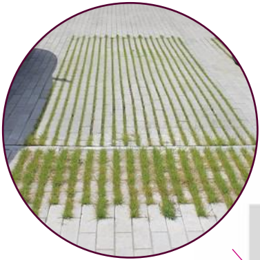
Parkeren in halfverharding
