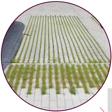
Parkeren in halfverharding
