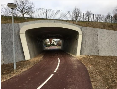
Fietstunnel MaasWaalpad (geopend in 2018)
