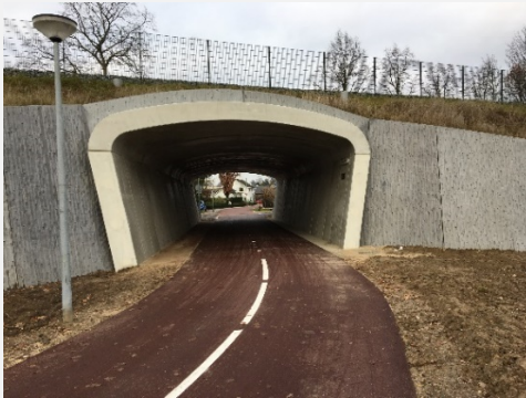
Fietstunnel MaasWaalpad (geopend in 2018)
