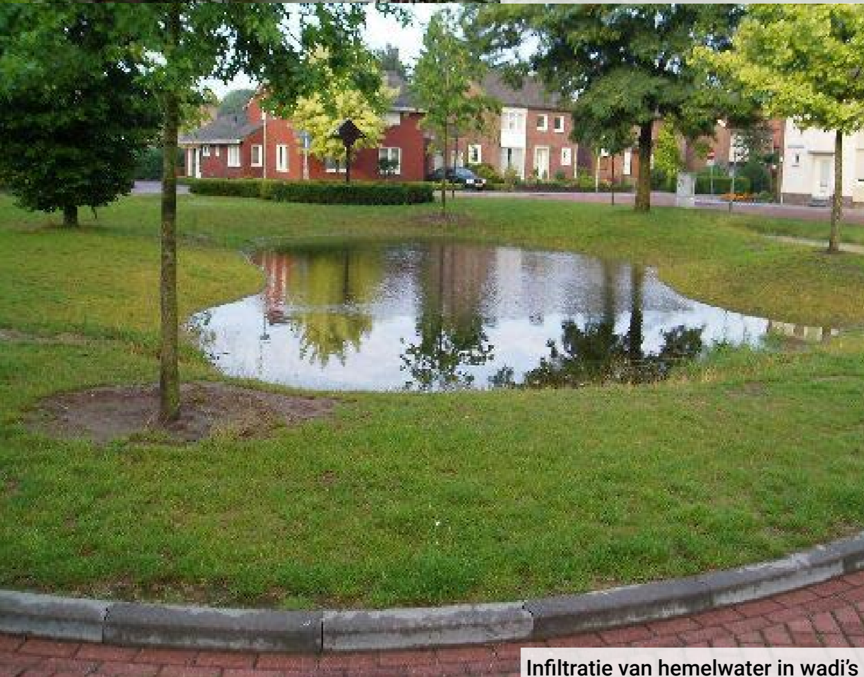
Infiltratie van hemelwater in wadi's
