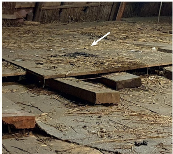
Figuur 8. Latrine steenmarter, 2 e verdieping.
