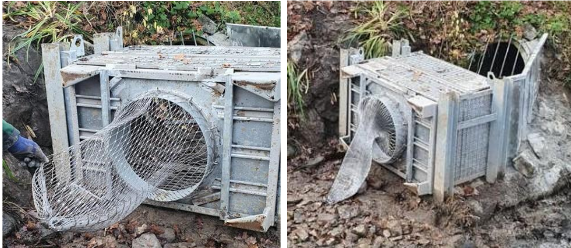
Figure 3 Dirtsocks that have been installed in Aachen
