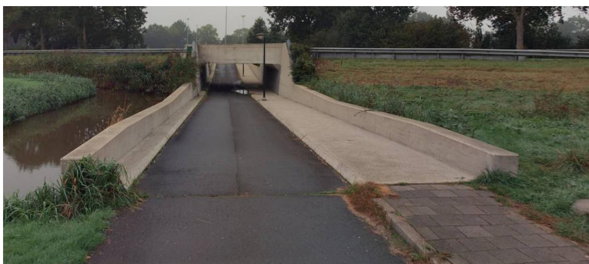
Figuur 23: Fietstunnel Hakkelbout, Nieuwkoop N231 ( https://streetsmart.cyclomedia.com )
