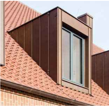
dakkapel oranjerode beplating
