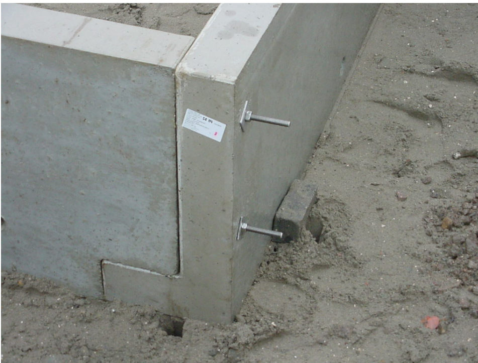
Detail boombunker
