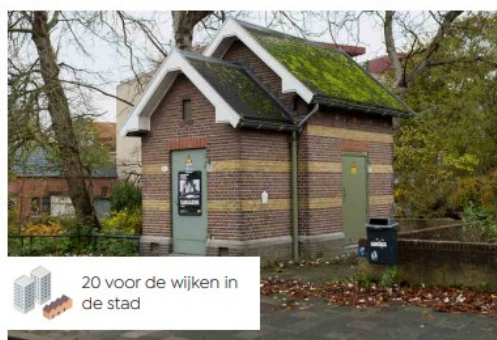
MS-MS station (3-23kV)
