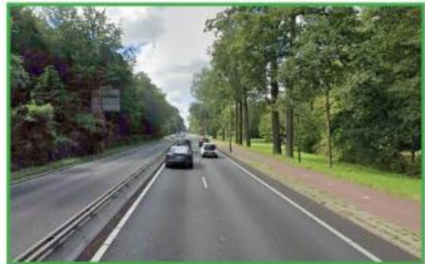
Figuur 13: Metalen barri re N44 (bron: Google Streetview)
