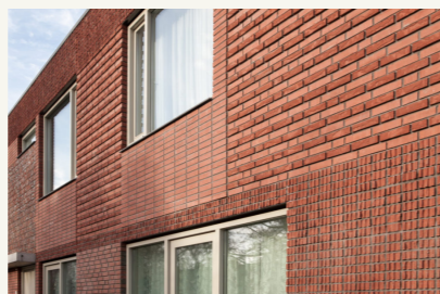
Detailering in metselwerk.
