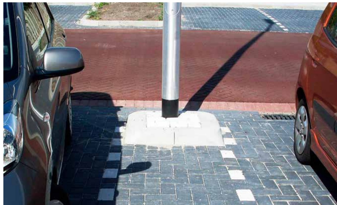
Lichtmast in parkeervak
